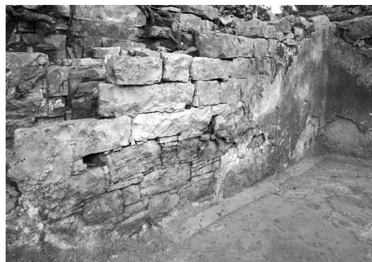
Fig. 1b. Detail of the northern corner showing drywall blocks as well as the multi-layered waterproof mortar
