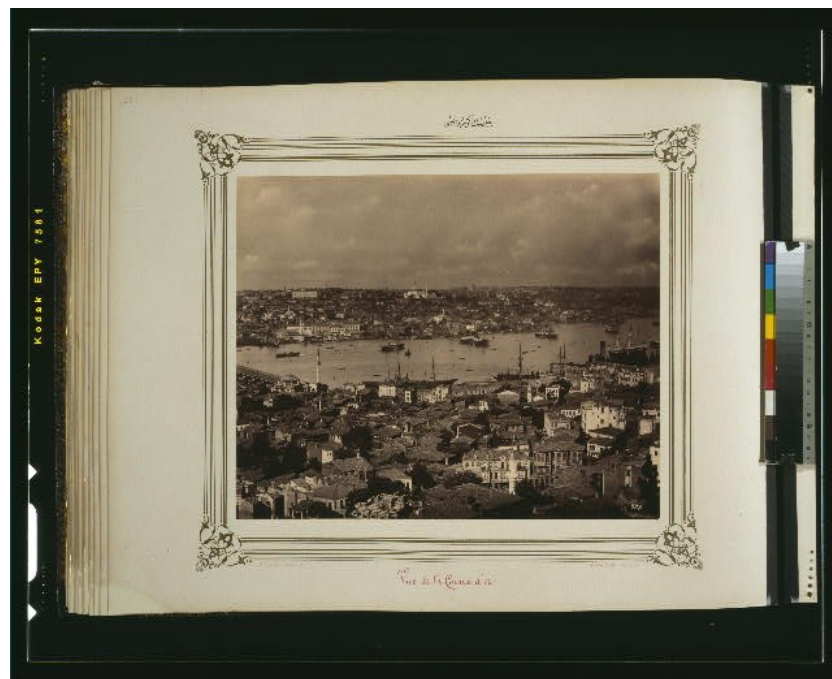
Slika 34: Pogled na Zlatni rog https://www.loc.gov/pictures/item/2003667954/resource/ . Pristup stranici: 20.4.2022.
