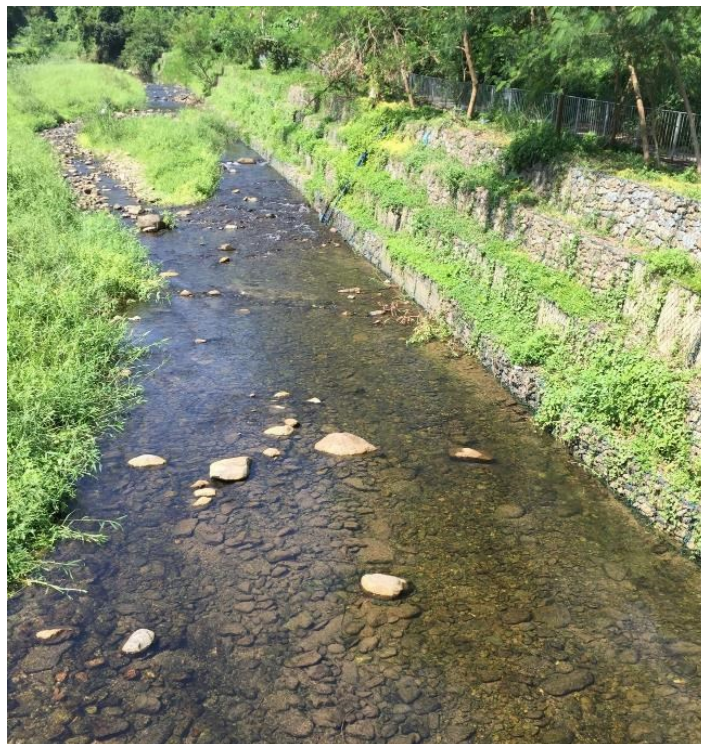
Sl. 43. Gabioni obrasli vegetacijom na jednoj strani korita gornjeg toka rijeke Lam Tsuen u Hong Kongu ( https://iwa-network.org/hong-kong-river-improvement-works-in-upper-lam-tsuen-river/ , pristup 22. 2. 2021.).
