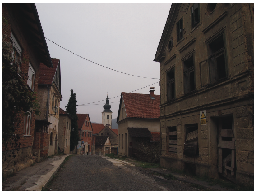
Figure 7. Empty and dilapidated houses in the center of the city of Hrvatska Kostajnica, Davorin Trstenjak Street (Region Pounje, Sisak-Moslavina County). Photographed by Sanja Lončar, 26. 11. 2020.
