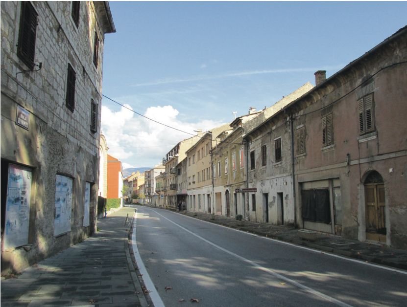
Figure 5. A series of empty buildings with residential and retail spaces in the center of the city of Knin, King Zvonimir Street (Region Dalmatian Hinterland, Zadar County). Photographed by Sanja Lončar, 8. 11. 2018.
