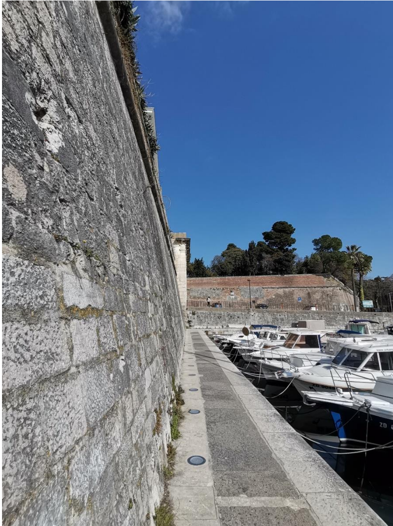
Figure 19. Zadar, view of the elongated Bastion Ponton and the corner of Porta Terraferma. Photographed by Karla Papeš.
